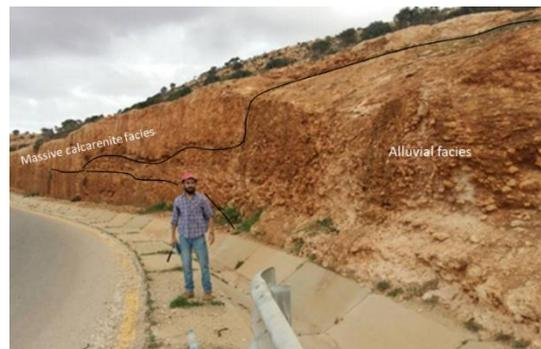
Fig. 9. Calcarenite beach deposits and alluvial deposits in Bersas Section
