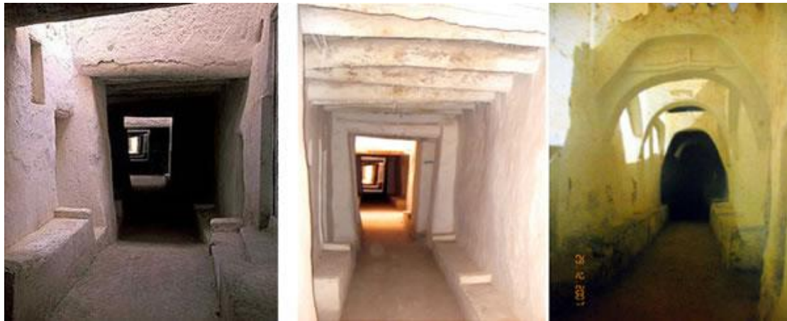
Figure 7: The covered walkways openings
