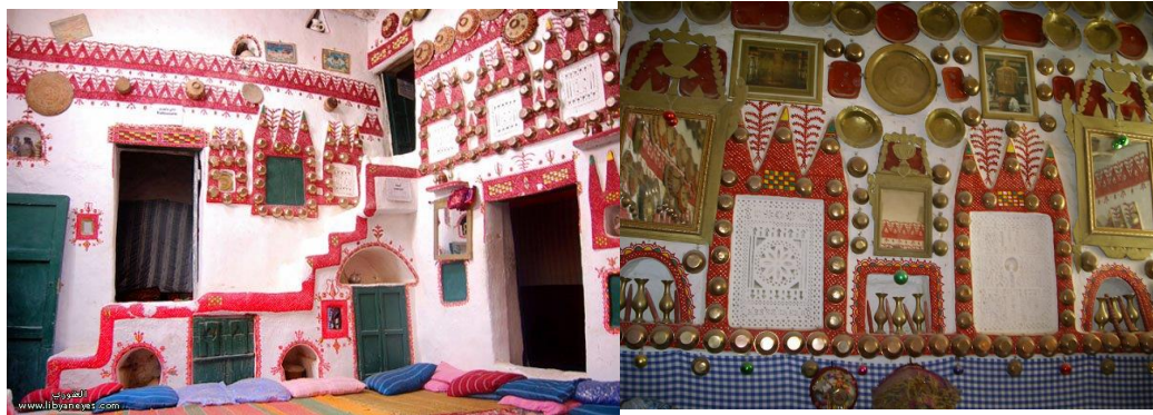
Figure 9: reflective mirrors and brass for daylighting efficiency
