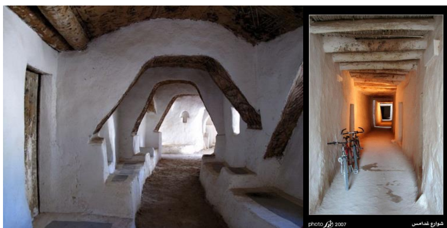
Figure 6: seating areas along the walk way
