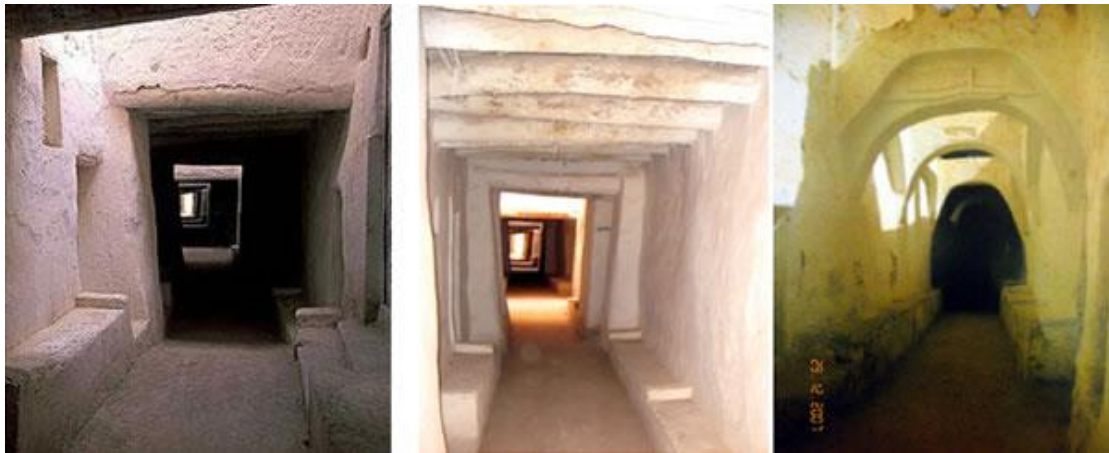
Figure 7: The covered walkways openings
